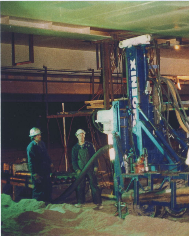
Figure 2: Work space under Molikpaq deck.
